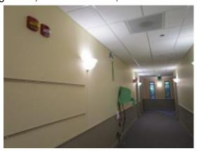
Corridors, restrooms and other common use areas were identified with a pair of horn/strobe devices installed inches from one another (see photo above). These devices should be installed every 50 feet, when placed this closely together they can cause photosensitive epilepsy. This risk is especially high for children and adolescents. These multiple devices were within the public circulation path in each location where this issue was identified.
